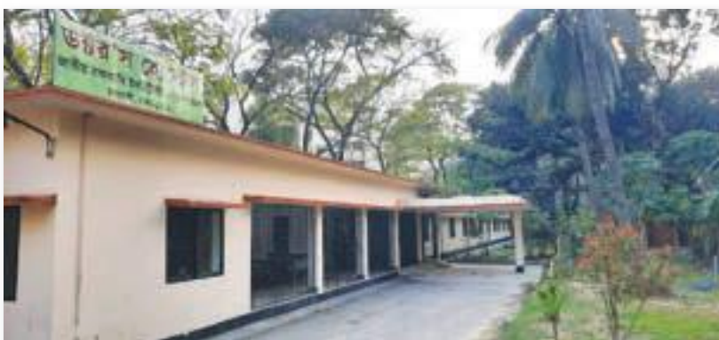
New renovated Doctors Hostel of NIDCH
